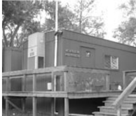
The KICA Maintenance offices are currently housed in trailers ranging from 15 to 25 years old.
